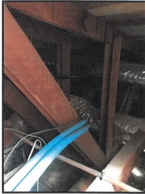
Partial West Roof Framing
