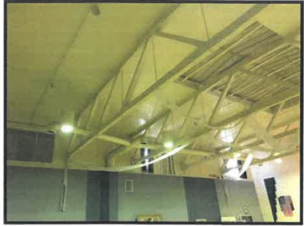
Interior Theater Roof
