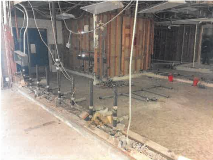
Remaining Plumbing Lines
