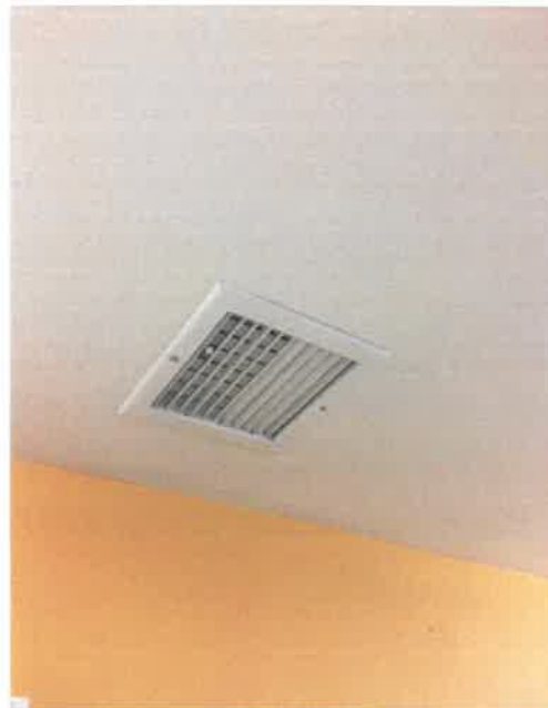
Typical Ceiling Register in hard lid
