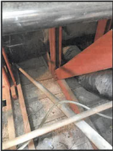
Partial West Roof Framing
