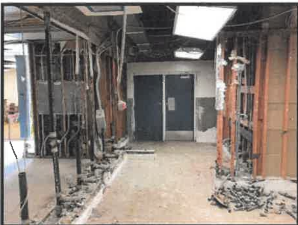
Photo 11 – Interior at Restrooms
