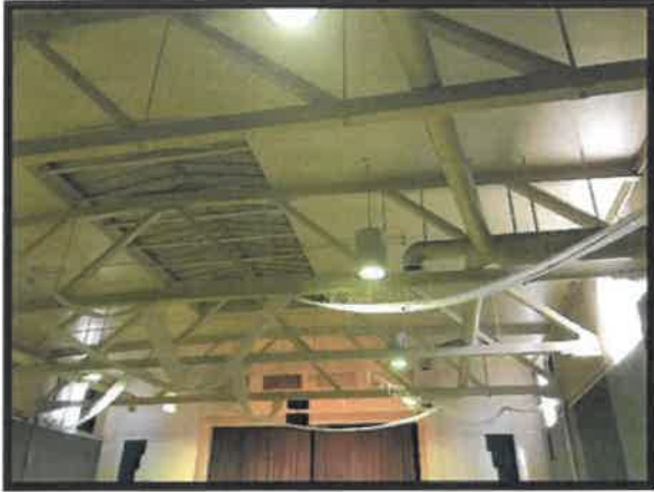
Interior Theater Roof
