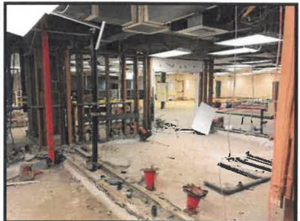
Photo 12 – Interior at Restrooms
