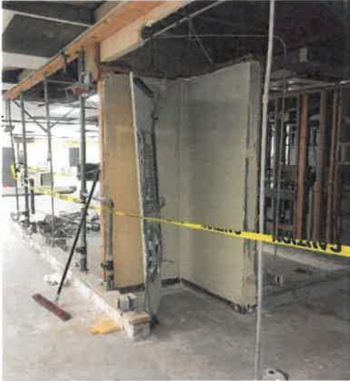
Existing Telephone Backboard
